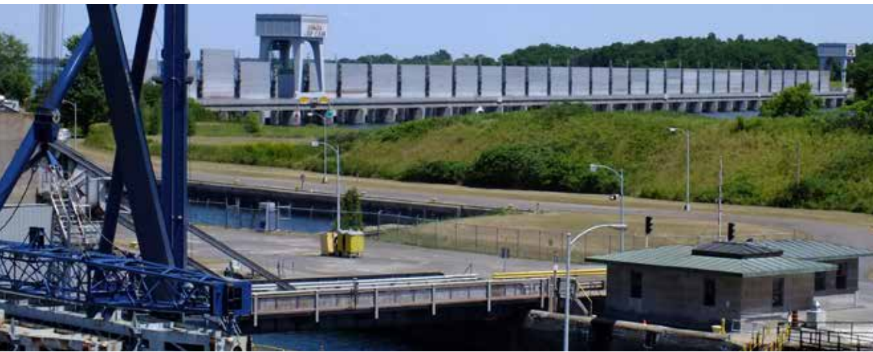
The Iroquois dam spans 603 metres across the St. Lawrence controlling water flow with 32 sluiceway gates.
