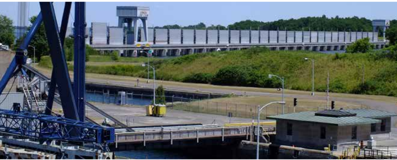
The Iroquois dam spans 603 metres across the St. Lawrence controlling water flow with 32 sluiceway gates.
