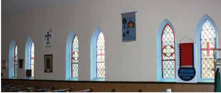
The diamond quarrel windows in St. Luke's Anglican Church, Lyndhurst, each with a central medallion
