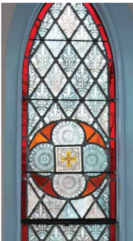
One of the original windows restored with pieces cannibalized from a single window
