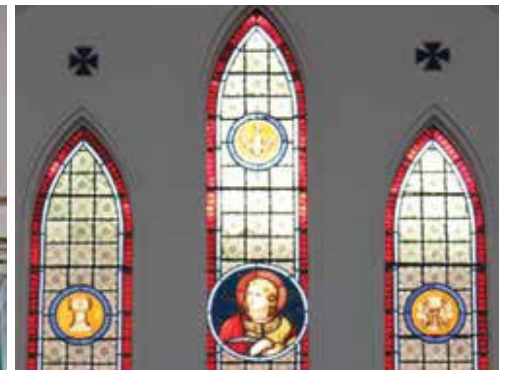
The altar window is a simplified triptych of square quarrel design with medallions
