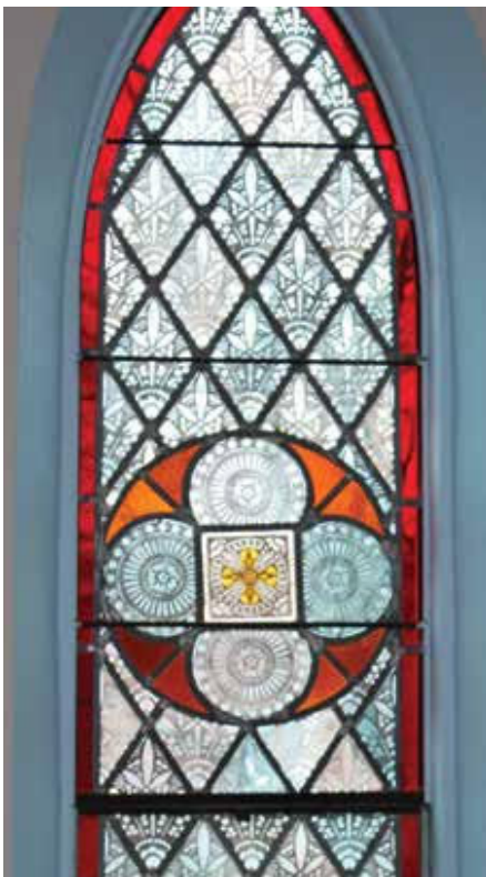
One of the original windows restored with pieces cannibalized from a single window
